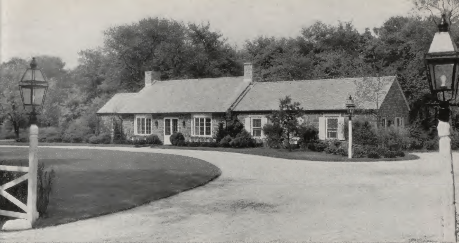
Above —The walls of Brook House, popular tea room near Brook Haven, Long Island, are dark colored concrete masonry. Units are laid up in a combination random and coursed ashlar pattern. Light colored mortar emphasizes the joints and the pattern. Aymar Embury II, architect. Leslie R. Marchant, builder.
